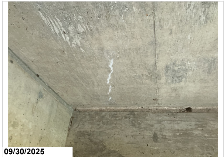
Span 1 Bay 3 efflorescence 3' CS2
