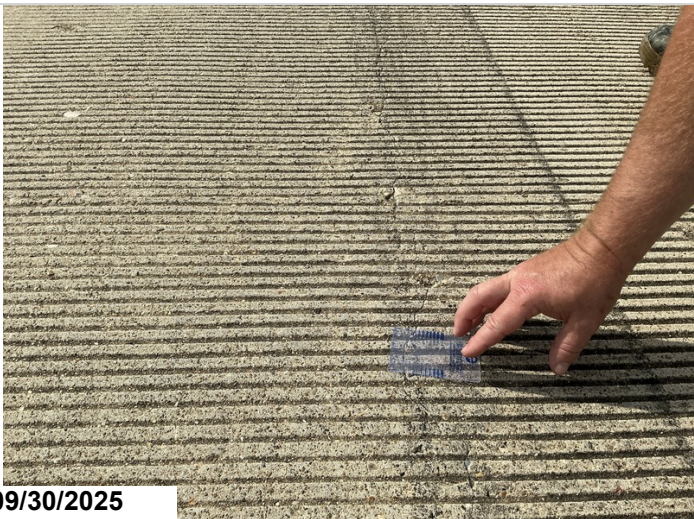
Span 7 longitudinal crack 35' up to 0.040"
