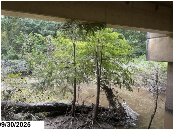
Span 4 right side trees growing under bridge
