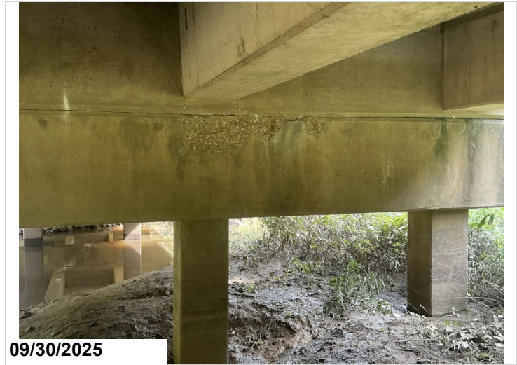
Bent 3 cap back spall 4' CS3
