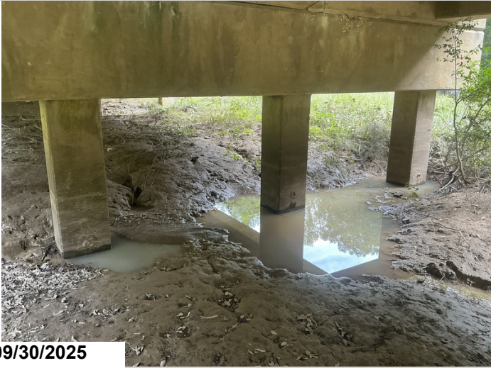
Bent 5 piles 2-4 local scour CS2
