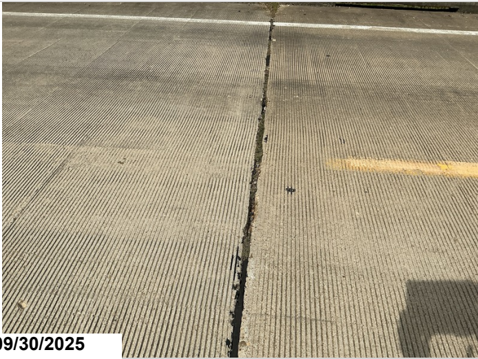
Bent 9 joint missing 9' CS4
